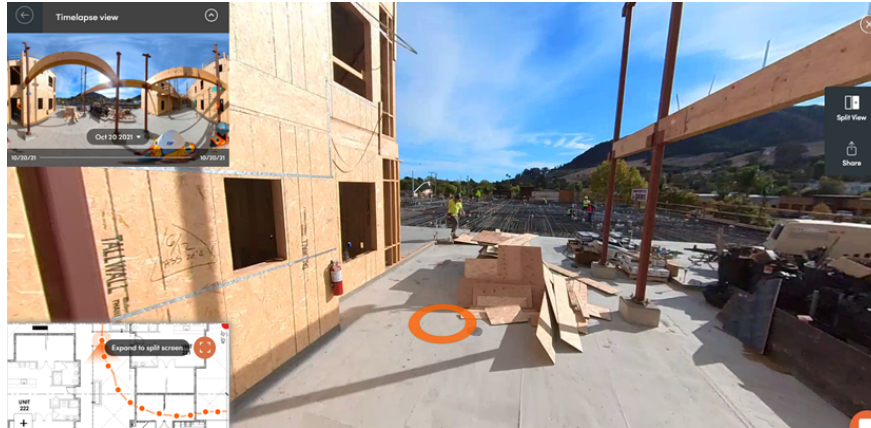
Figure 3. StructionSite, Inc. VFT Walkthrough Visual Example
