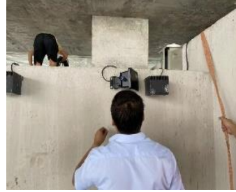
(b) The Radar of Deflection Monitoring
