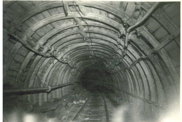
Fig. 8. An example of good stability of a roadway driven in compacted and consolidated goaf
